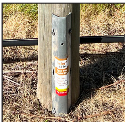
Ocloc half post repaired with Ocloc V
